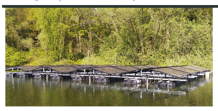
DC Solar Systems introduces the FloatFix mounting system, suitable for inland waterways such as water basins and sand excavations. The system is modular, easy to install and ensures that sufficient air and light can still reach the water. This preserves water quality and cools the panels properly, reducing the risk of overheating while producing more power, and ensuring the panels last longer.
