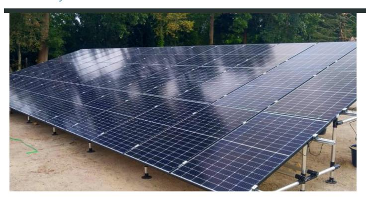
DC Solar Systems introduces FlexFix Ground, the flexible mounting system for ground-mounted solar systems. There are two options, one based on ground columns, which can easily be placed in the ground. The other is based on ballast tubs, in case placing a column into the ground is not possible. Both systems can be mounted without heavy installation equipment, ensuring minimal disturbance of the soil.
